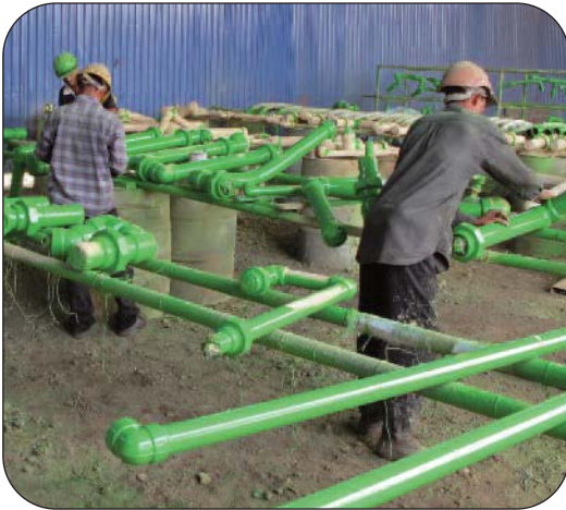
Thorburn Malaysia rigid pipe final assembly before packaging
